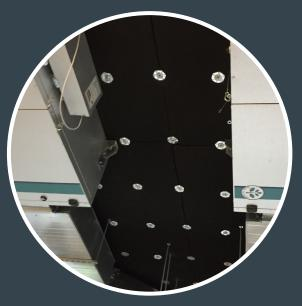
Pyrosorb is specified as a high performance acoustic barrier between walls and floors as pictured here – 25mm self-adhesive backed sheets adhered and fixed to concrete soffits between floors
